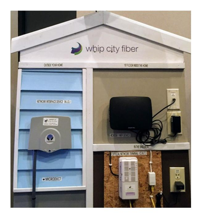
Images showing samples of equipment. The exterior Network Interface Device on the left is 8.6" wide by 7.3" tall. The Optical Network Terminal in the bottom right is about 3" wide by 6" tall, and is usually wall-mounted in a basement location. The WiFi router in the top right is about 8" wide by 7" tall, and is usually located in the center of the first floor to provide the best WiFi signal throughout the home.
